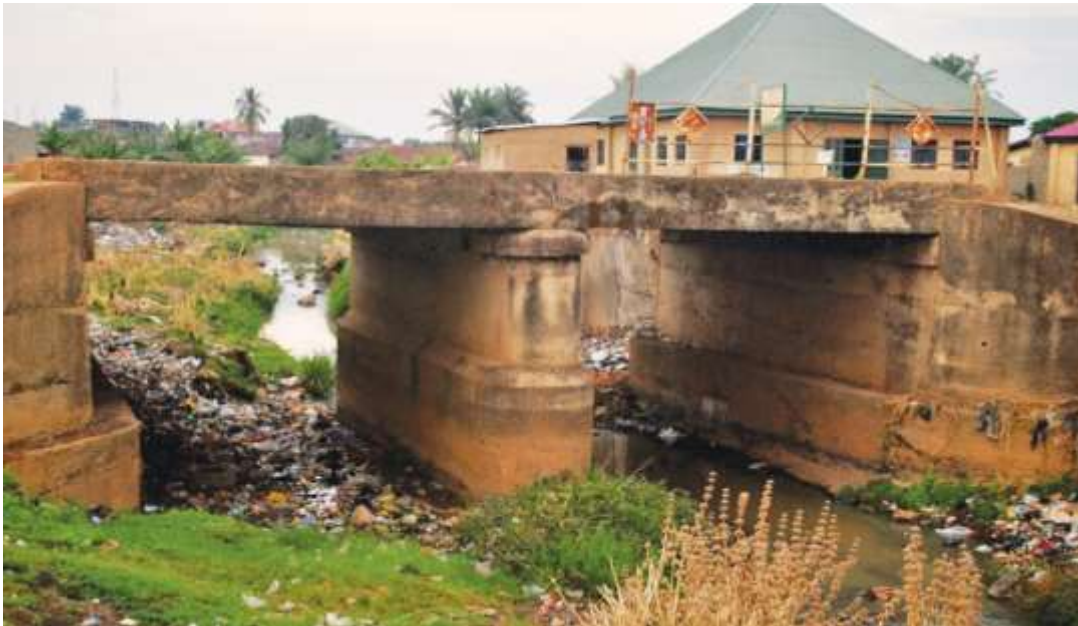
Image 2: Takau bridge in Jema'a Kaduna
