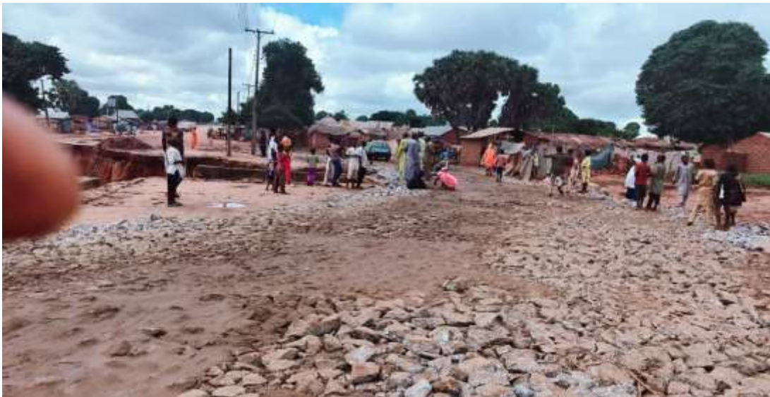
Plate II: Rehabilitated road in Rafin Gora
