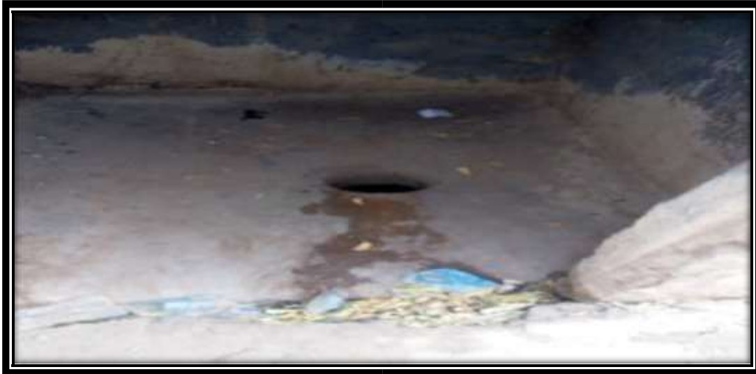
Plate VII: Birniwa Pit Latrine Evacuated, for Bioremediation to a Farm.
