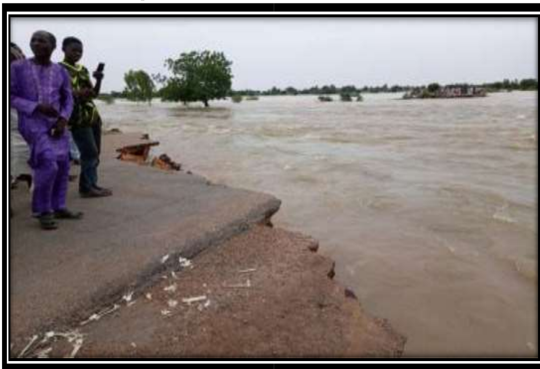
Plate 1 Picture of the Collapsed Hadejia Road
