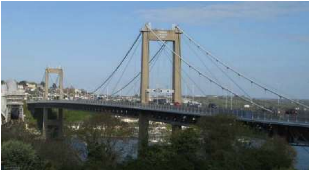
Figure 1.0: Tamar suspension bridge
