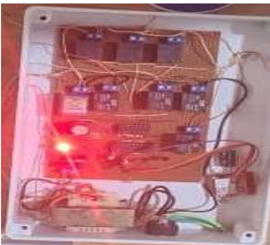
Figure 10 The Internal Picture of the Designed System
