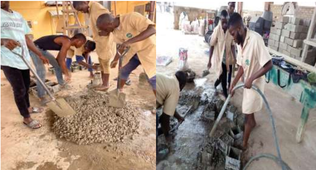
Plate 1 : Mixing of concrete
