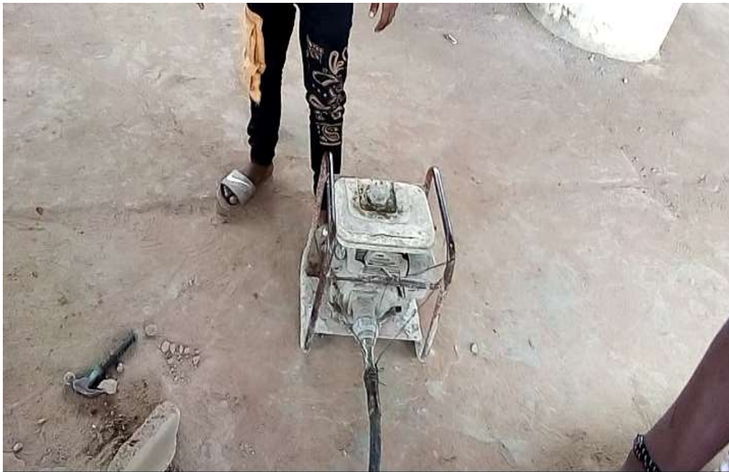
Plate 4 : Concrete Vibrating Machine
